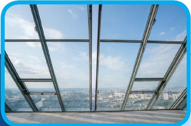
Electric heating can even be installed in moving glass panes, such as these sliding doors measuring 6.5 meters in height and 12 in width at Mercury City Tower's penthouse
